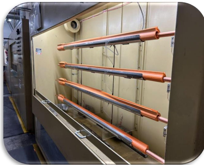
Figure 2 - Line Hose Dielectric Testing
